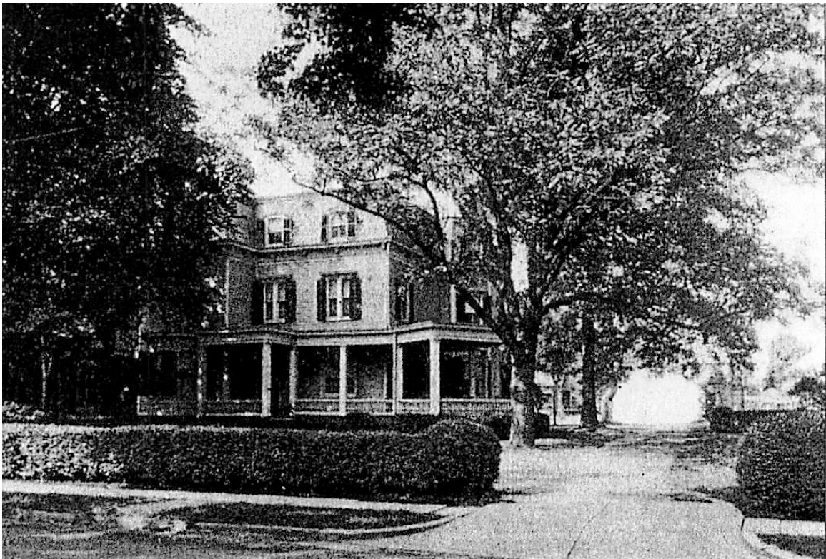
40-42 Washington Avenue, former H.R. Munger House ca. 1872, was demolished just a few years ago
