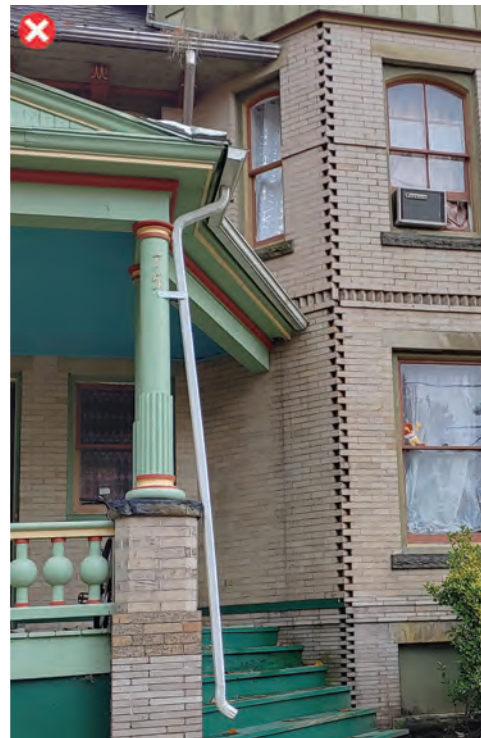
Downspout placement outside of cornice
