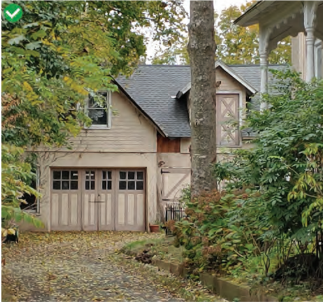
Well-maintained original carriage house
