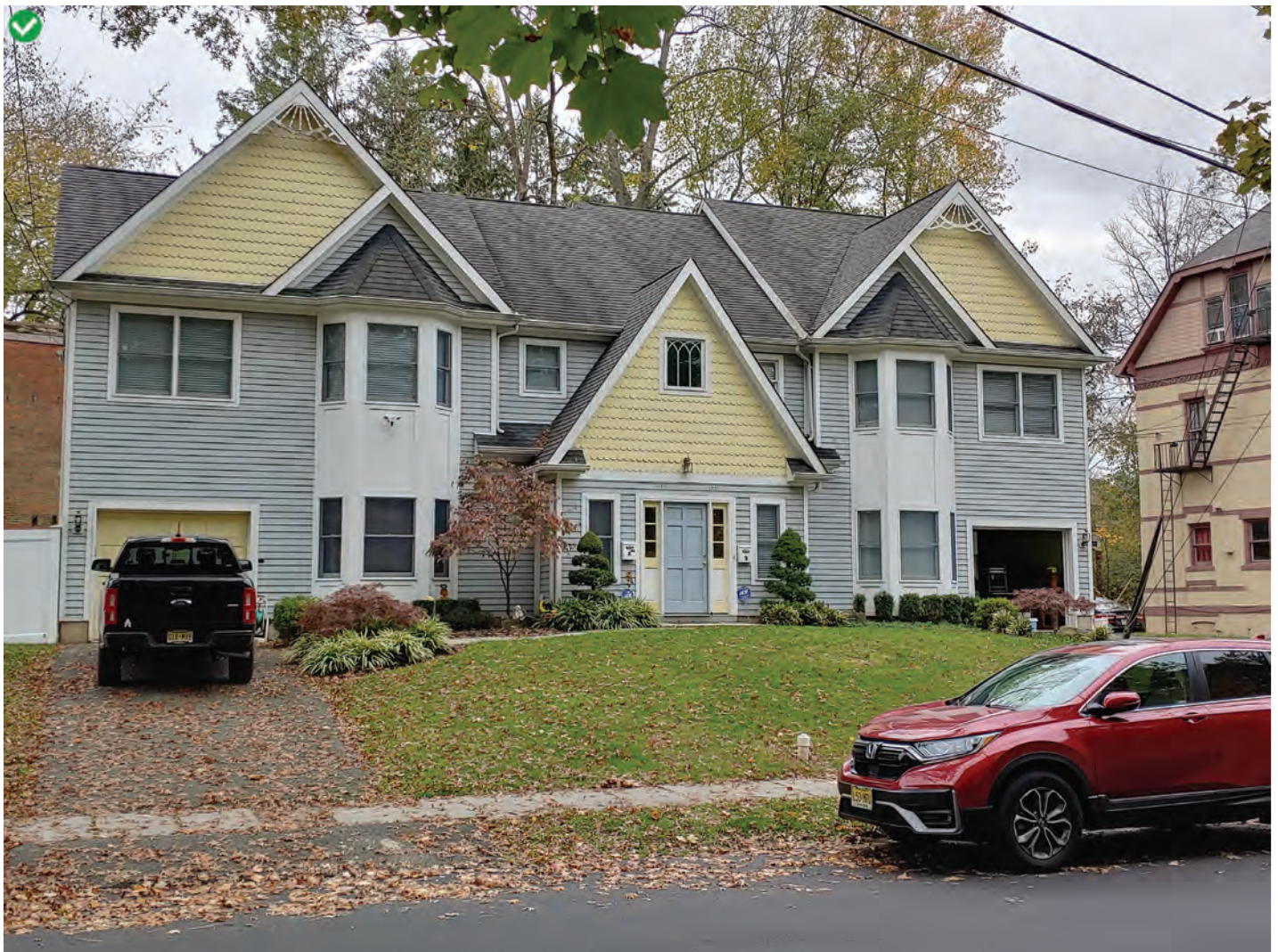
New construction on Sycamore Avenue that alludes to the scale and design styles, such as wood siding, of the neighborhood while remaining visibly contemporary.
