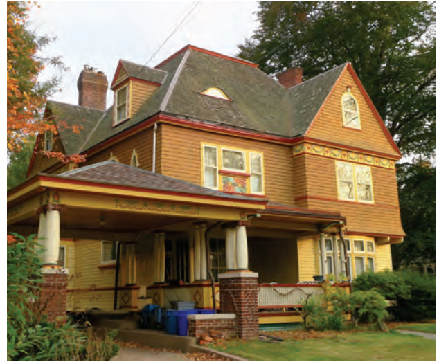
Asphalt shingle hipped roof with dormers
