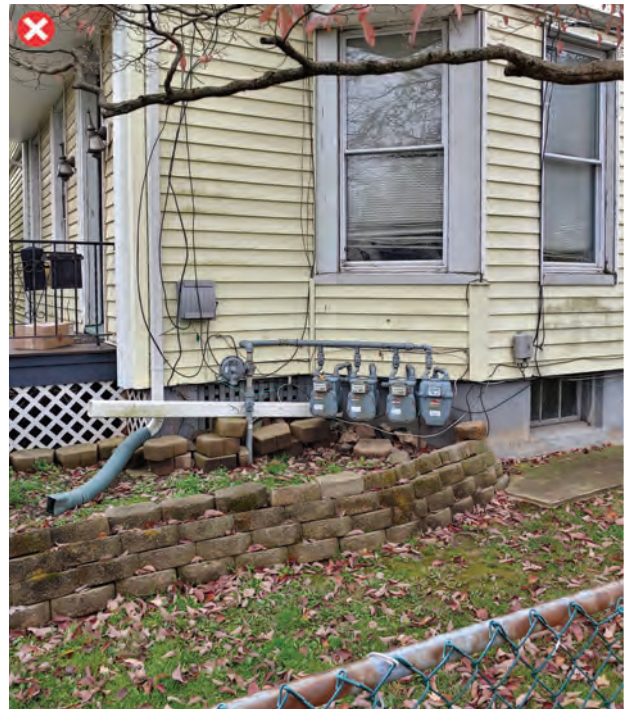
Incompatible stone block retaining wall in front yard
