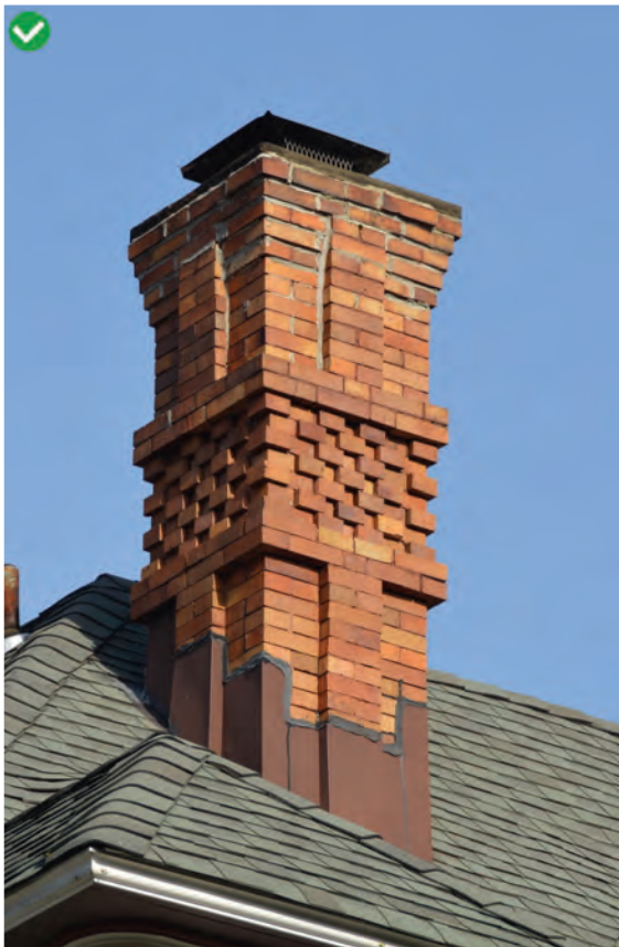
Decorative brickwork chimney that has been maintained with flashing installed correctly
