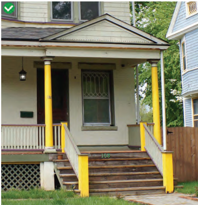
Appropriate matching wood railing and stairs
