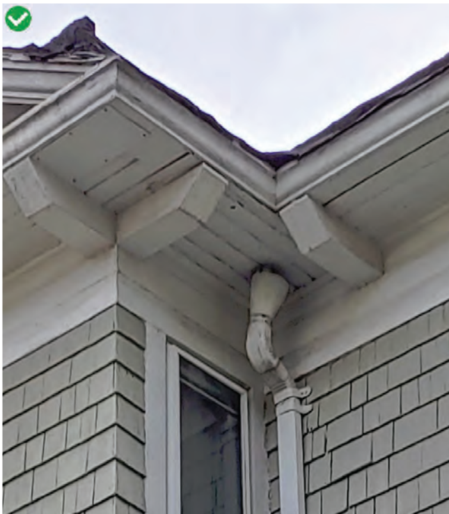
Downspout placement underneath roof fascia
