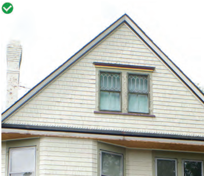
Original lead came windows intact and maintained
