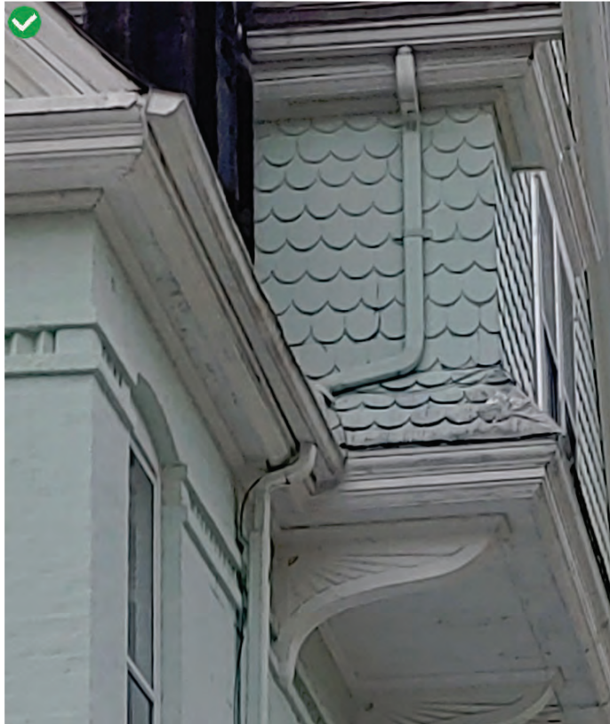
Downspout is concealed and matches shingle paint.
