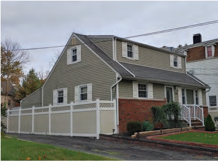
Asphalt shingle side-gable with dormer
