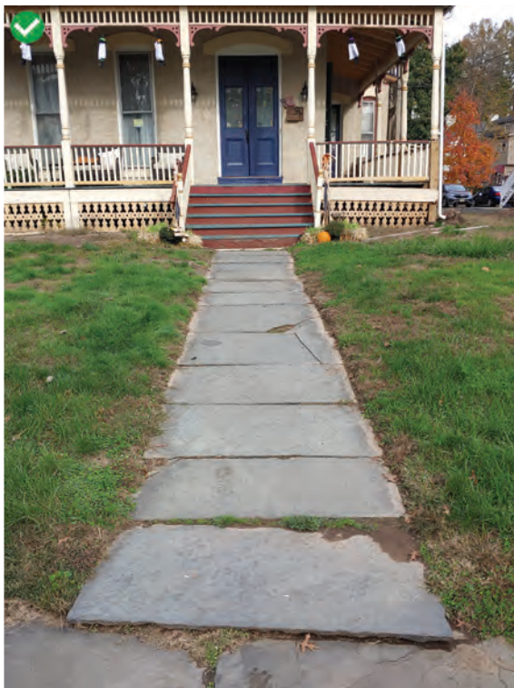
Historically compatible flagstone walkway
