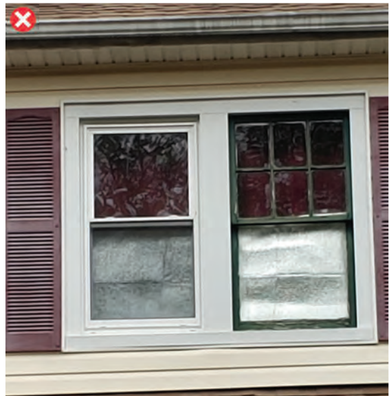
Replacement aluminum window (left) and original wood window (right)
