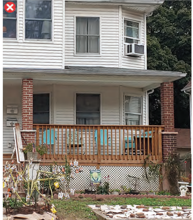
Air conditioning unit on street-facing elevation
