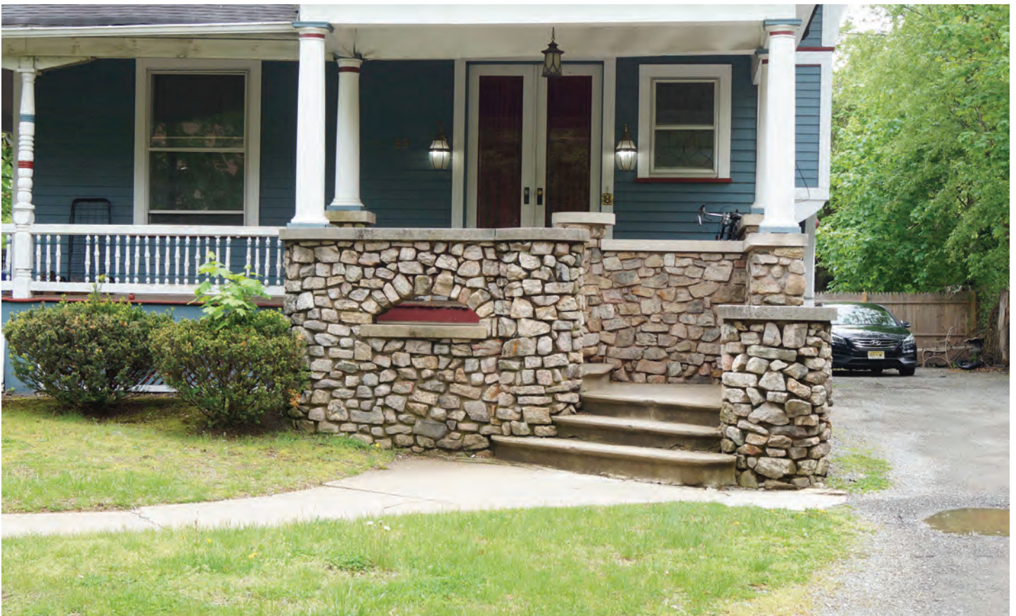
Stone porch on Willow Avenue
