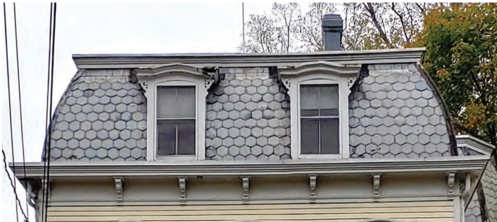
Convex mansard with slate shingles
