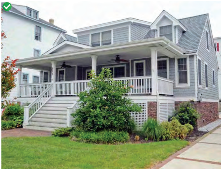
This house incorporates brick with flood vents and lattice panels, both appropriate for the architectural style. Photo from NJHPO Elevation Design Guidelines
