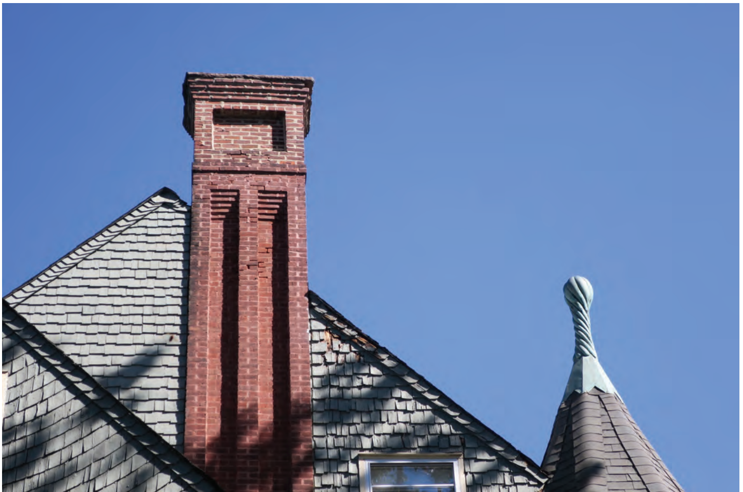
Mercer Avenue residence with wooded shingle roof and decorative masonry chimney
