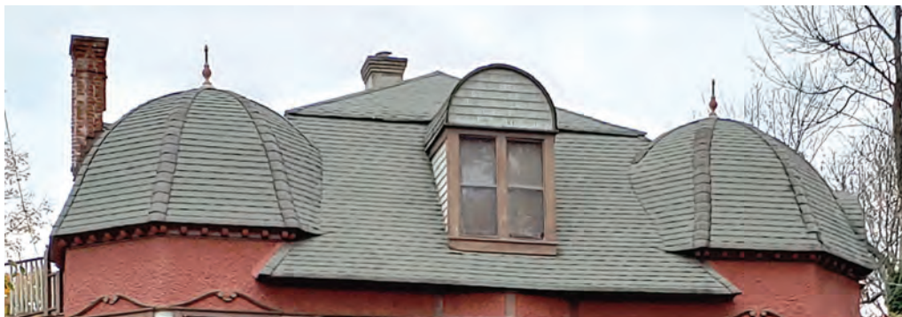
Asphalt shingle roof with towers and dormers
