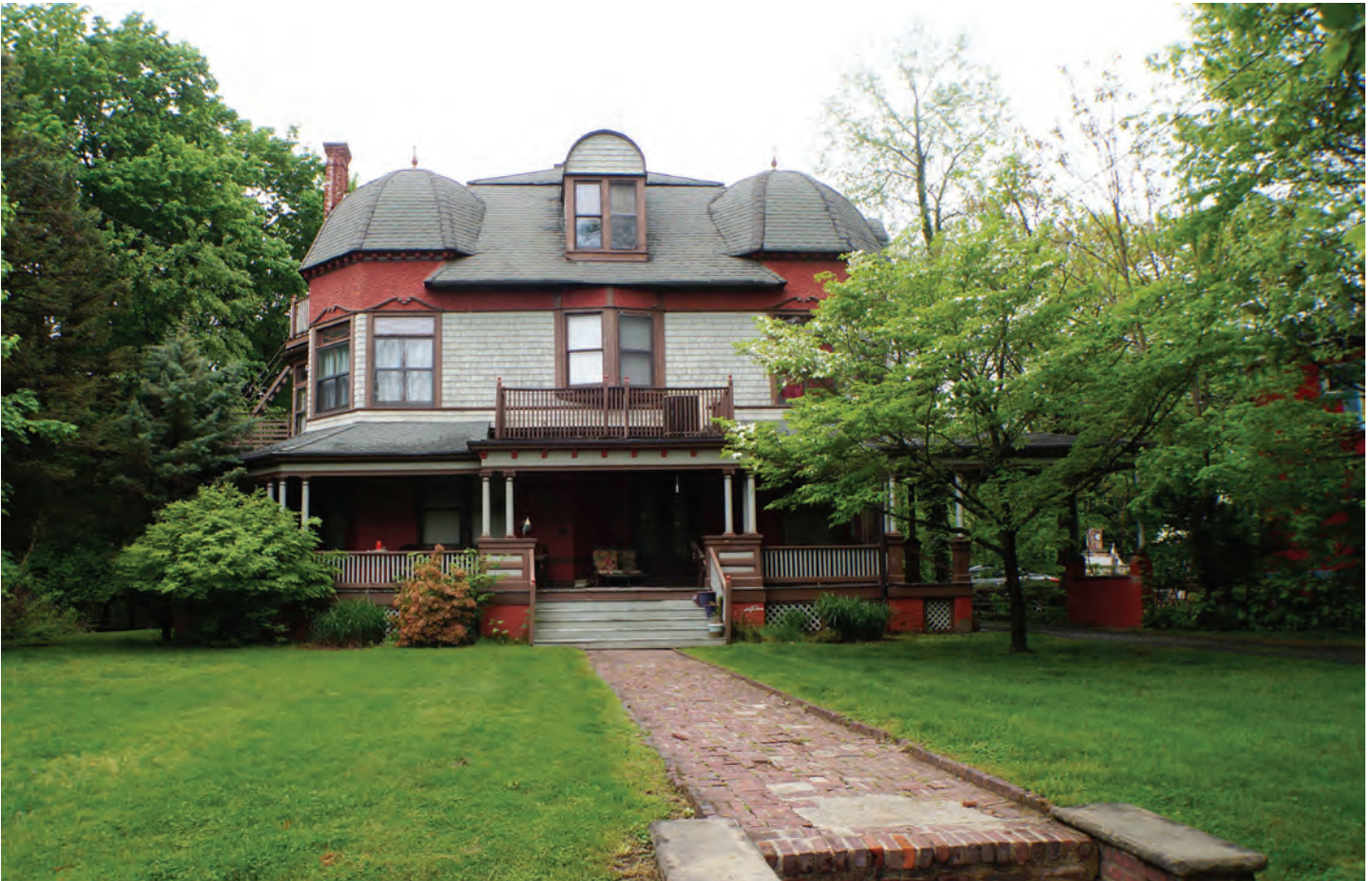
Rockview Avenue residence with historic brick walkway. Repairs to damaged areas should be made with in kind material
