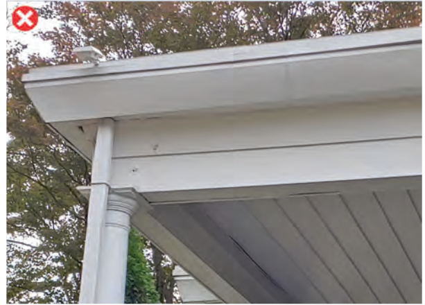
Vinyl porch ceiling with attached floodlights
