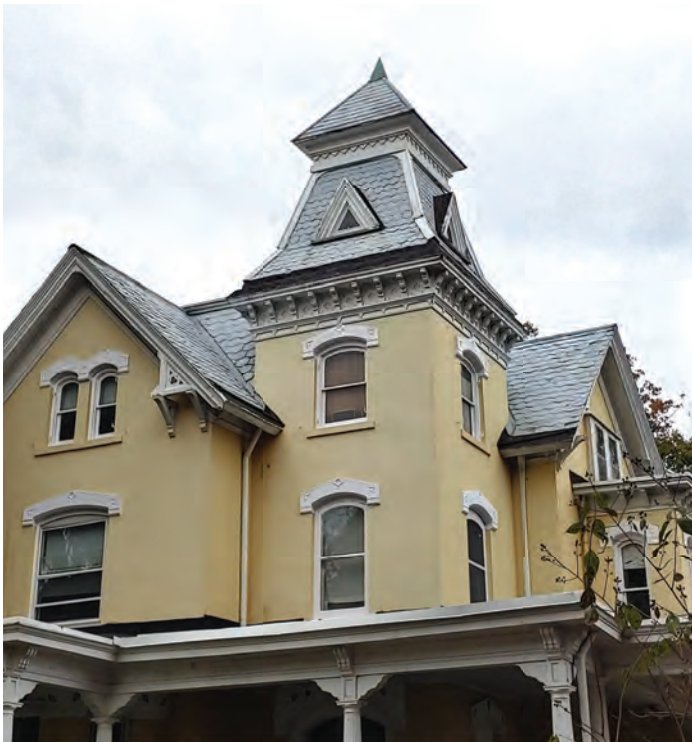
Asphalt shingle cross-gable with tower
