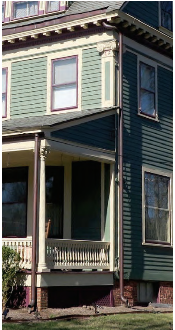
Historical gutter system on Myrtle Avenue residence
