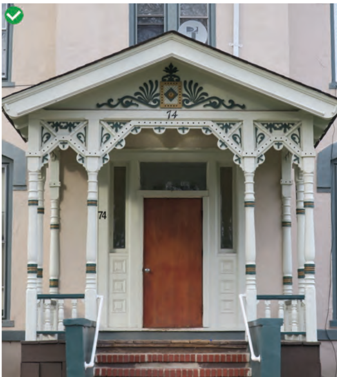
Original ornamental features are preserved and maintained
