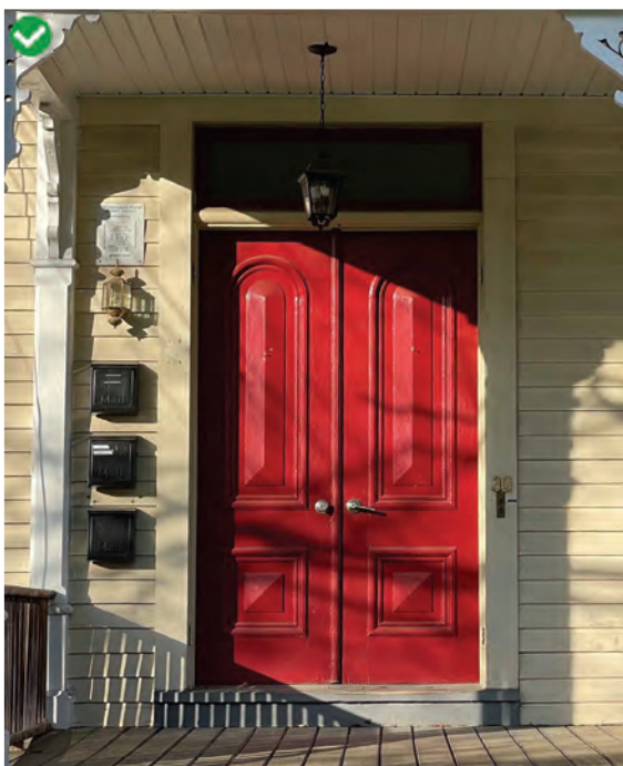
Maintained original wood door and transom
