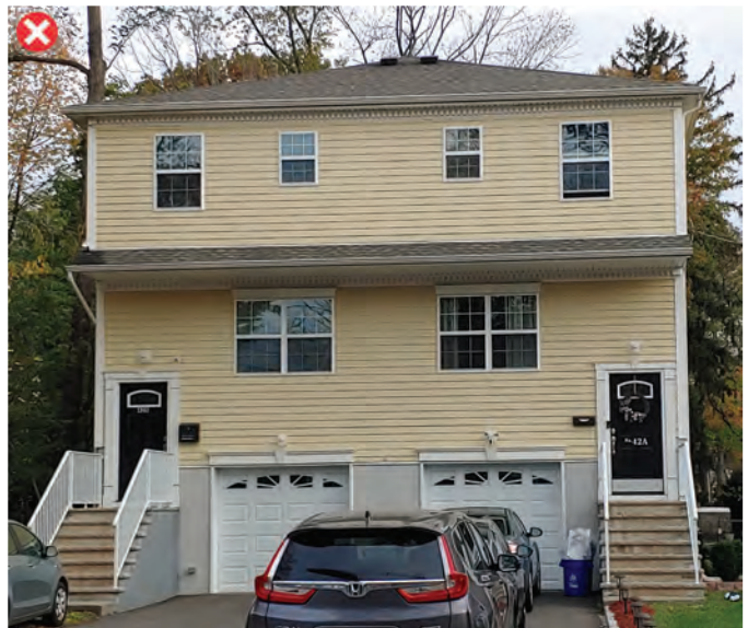
New construction with historically incompatible attached garages
