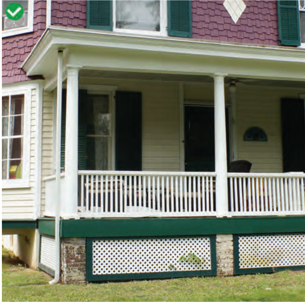
Appropriate railing and wood lattice
