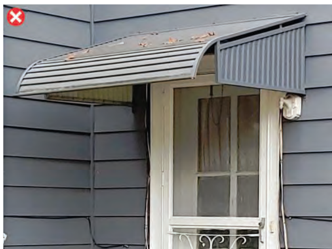
Sheet metal awning
