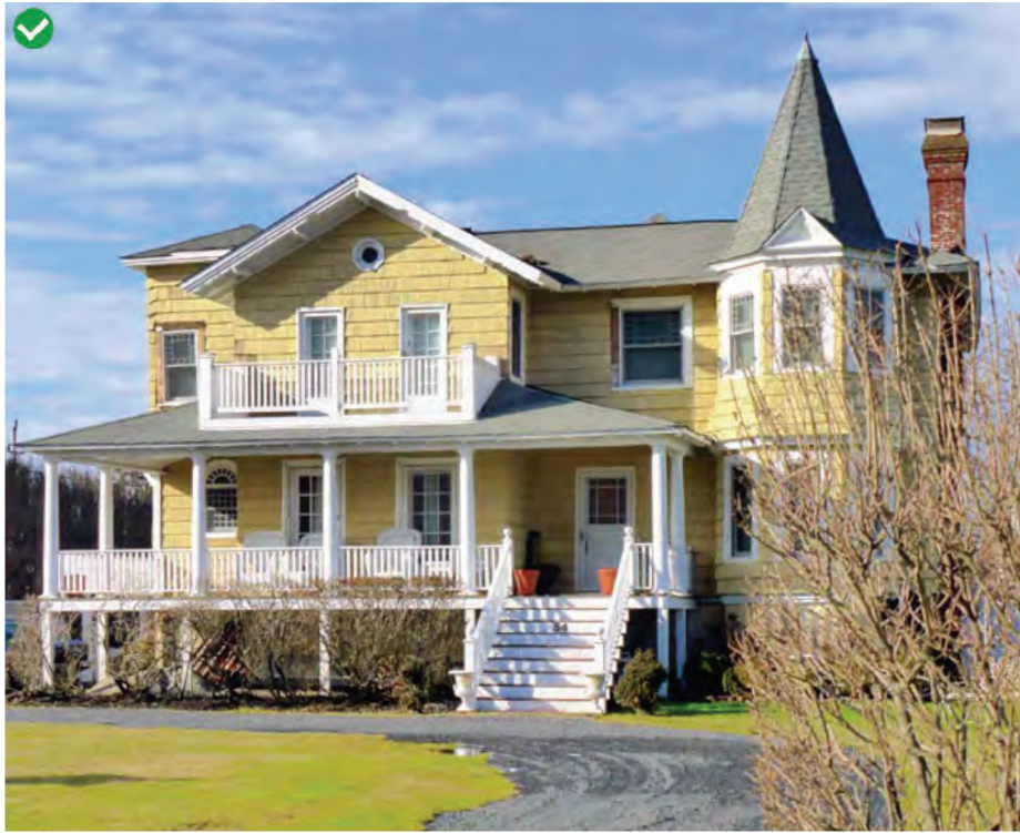
This house retains defining architectural features, and shrubs conceal raised porch. Photo from NJHPO Elevation Design Guidelines
