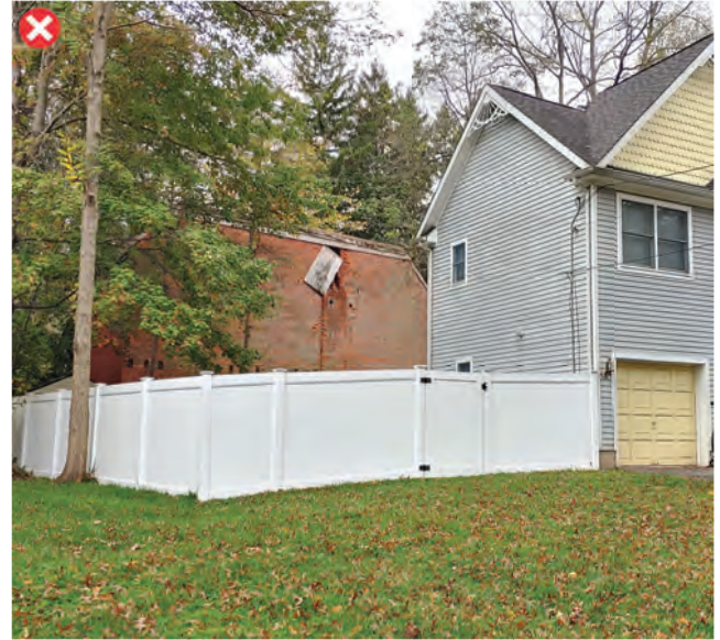
Incompatible vinyl privacy fence
