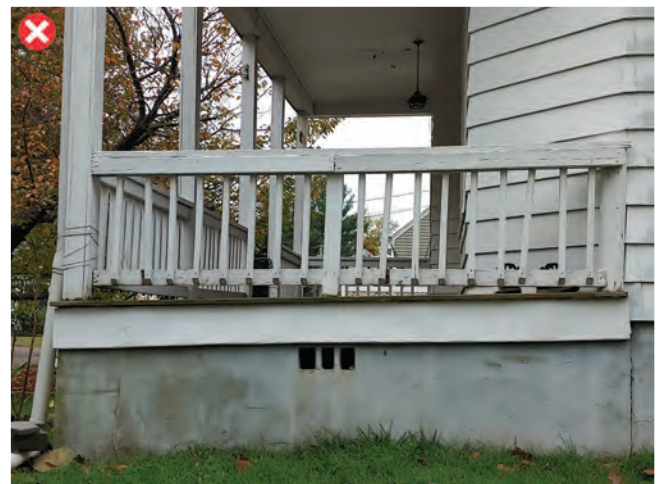
Foundation infilled with concrete block
