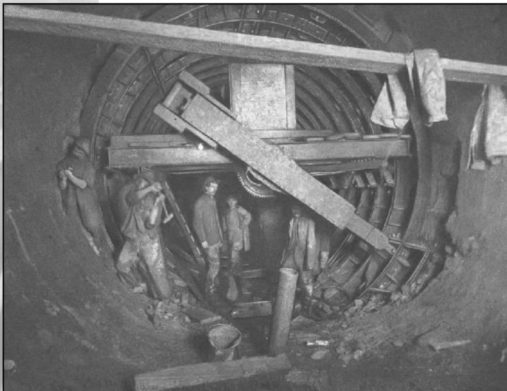
The existing Hudson River tunnels were completed in 1910.
